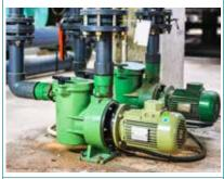
a system that maintains circulation of water through a public spa by pumps, and that provides continuous treatment that includes filtration and chlorination or bromination and any other process that may be necessary for the treatment of the water
