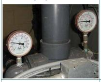
• two gauges are located on the top of the filter tank; one measures the amount of water flowing into the tank and one measure how much flows out of the tank. When too much dirt collects in the filter medium, the water flow rate drops. The difference is indicated on the gauges. If you notice a difference between the gauges, consult or refer to the manufacturers directions as filters vary in backwashing and pressure requirements.
